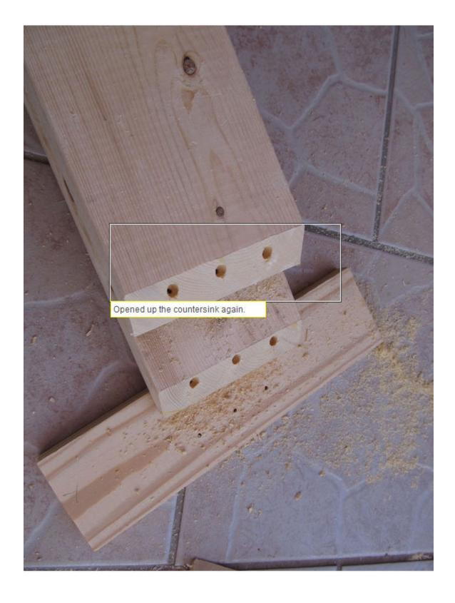
I'm a big fan of pre-drilling, so I started on the end pieces. I figured two screws into each end of the 2x4 ought to be sufficient. So, after a few quick measurements I drilled those holes. Then I pre-drilled the wood for the joints at the 4 corners.
