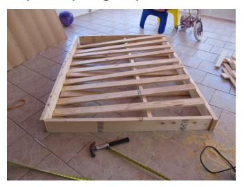
Measurements ready, I decided to make the longest sides of the bed the full length (79"). The shorter pieces would fit inside. The width of the frame is 59.5". Take away 1.5 from each side for the 2x6's and the cross pieces are 56.5" in length. The 2x4 center support is 79" less 3" from the front and back of the bed for a length of 76".
